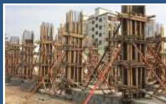
Shuttering Works
